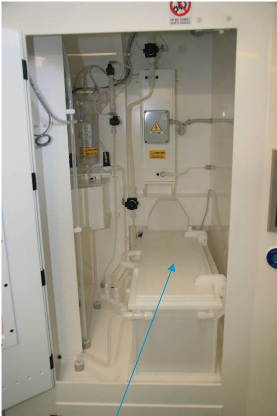
HI density PE tank with manual cover
