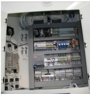
General control with Ormon PLC and SMC valves
