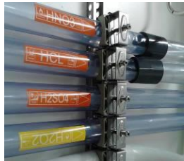
Double or triple piping lines installation and test
